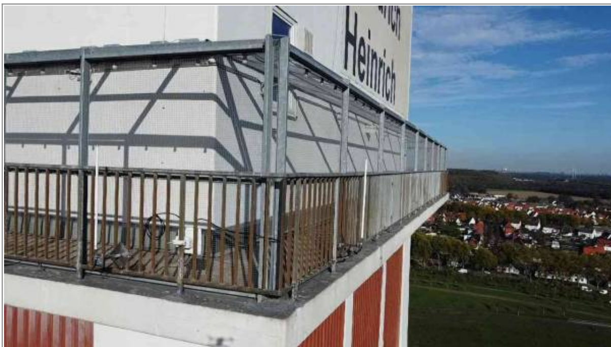
Fig.: The two rod antennas at the southwest corner of the tower of the former Friedrich-Heinrich colliery.
