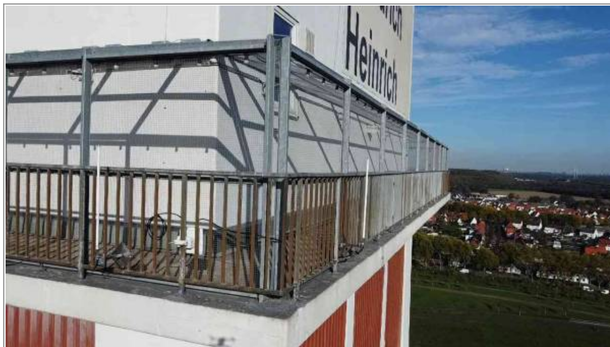
Fig.: The two white rod antennas at the southwest corner of the tower of the Friedrich-Heinrich colliery.
