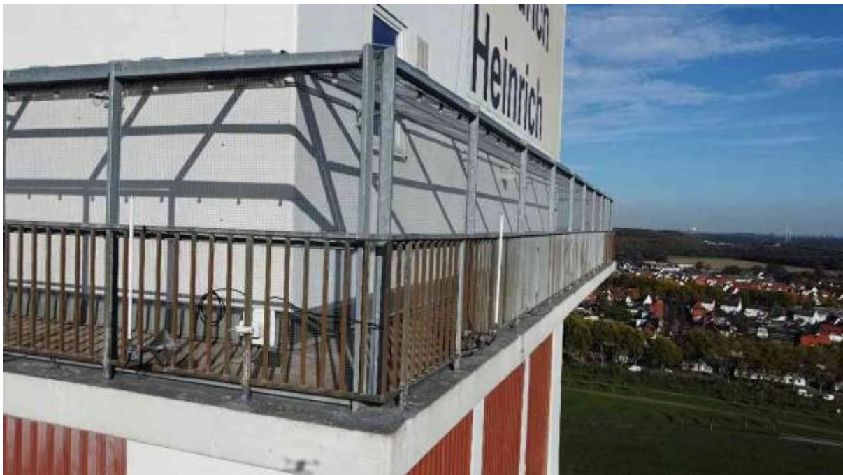
Fig. 1: The two white rod antennas at the southwest corner of the tower of the Friedrich-Heinrich colliery.
