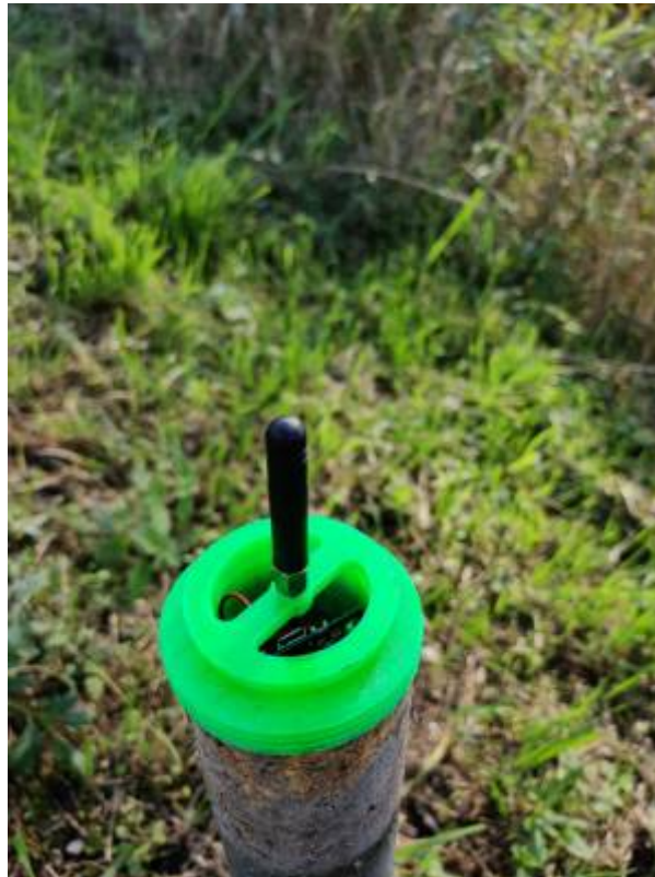
Fig. 1: Sensor and LoRa-Sender installed in a pipe without cover
